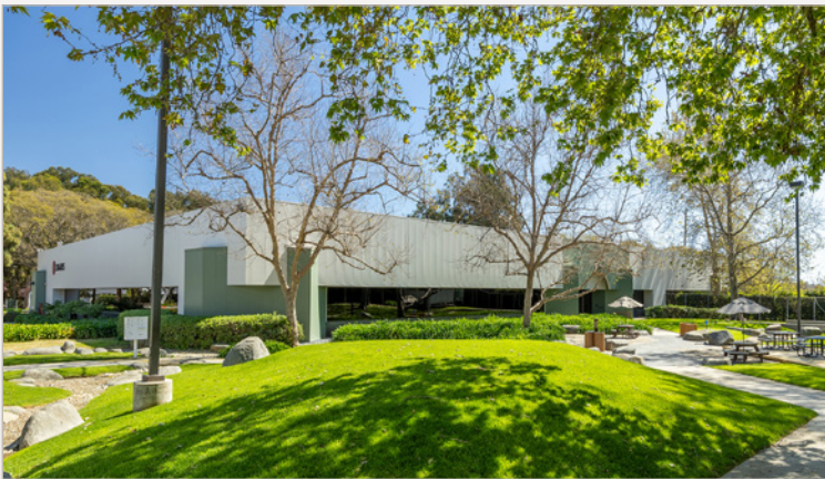
7414 Hollister Ave is a 40,487 SF creative office building leased by Umbra Space in Q2.
