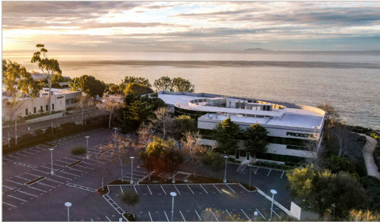
PlanMember Services leased 42,395 SF at 6267 Carpinteria Ave, previously occupied by Procore.
