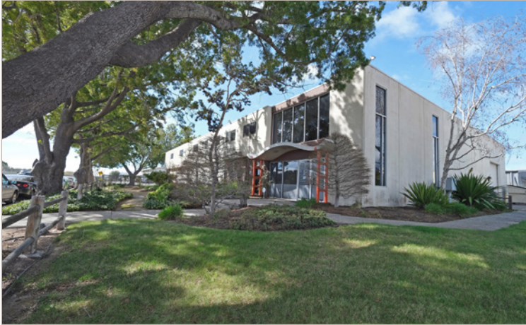
801 S Kellogg Ave in Goleta was purchased by an owner-user in Q4, which proved to be the largest industrial sale of the year.
