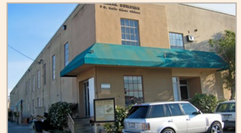
1 N Calle Cesar Chavez, Santa Barbara 11,845 sf – US Air Conditioning
