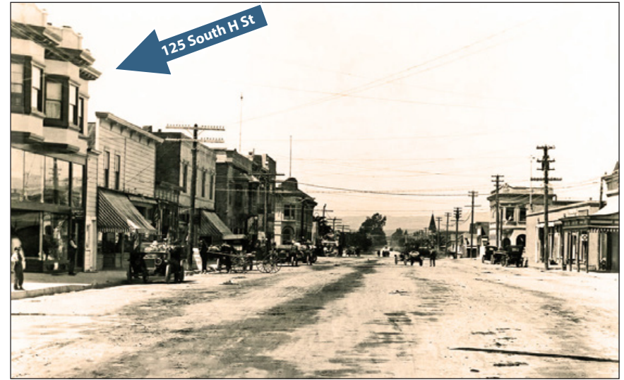
The new J.C. Long Building overlooks South H Street, 1910s
