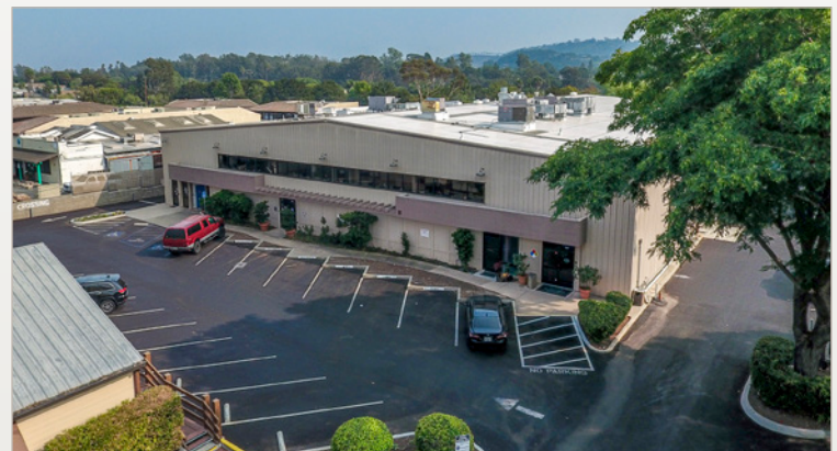
4183 State St is fully leased after Katz-Moses Tools signed 15,674 SF with 5,000 SF sublessee Spracher Engineering in tow.
