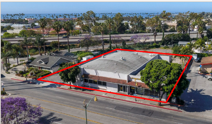
The 7,386 SF Retail/Industrial building at 18 S Milpas St in Santa Barbara was leased for 15 years by Aqua-Flo Supply.
