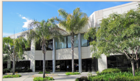
5425 Hollister Ave, Goleta 17,920 SF – Cottage Health
