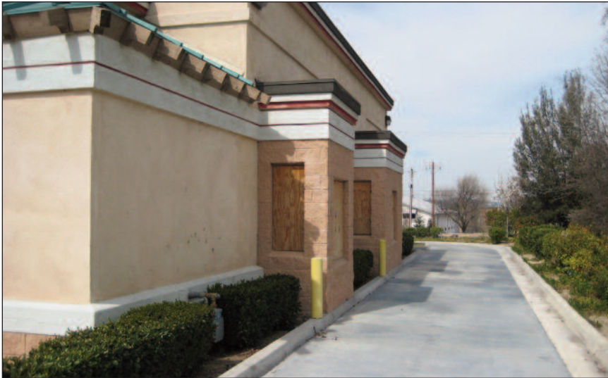
Double Window Drive-Thru Lane
